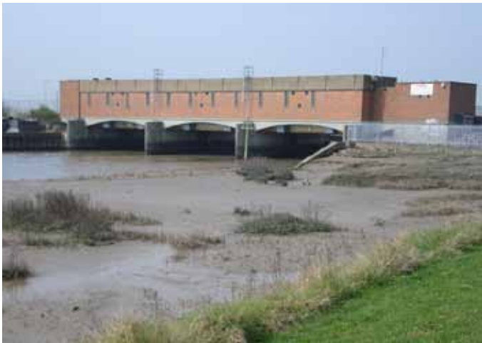
Flood barrier on Benfleet Creek © Jenny Lunn
