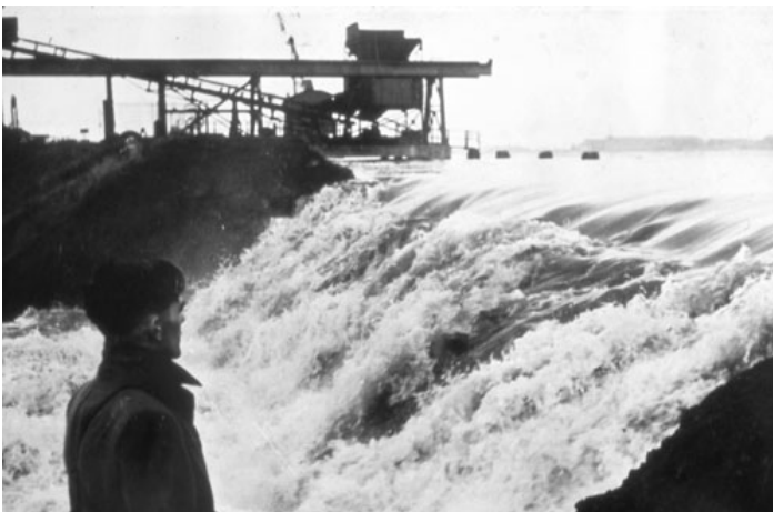
A breach at Erith during the 1953 floods Wikimedia Commons (CCL)
